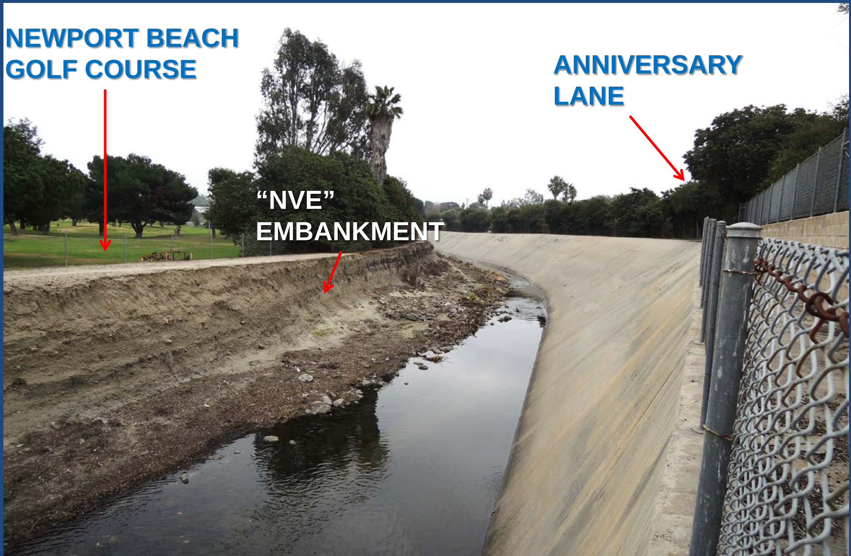
View Looking Downstream
