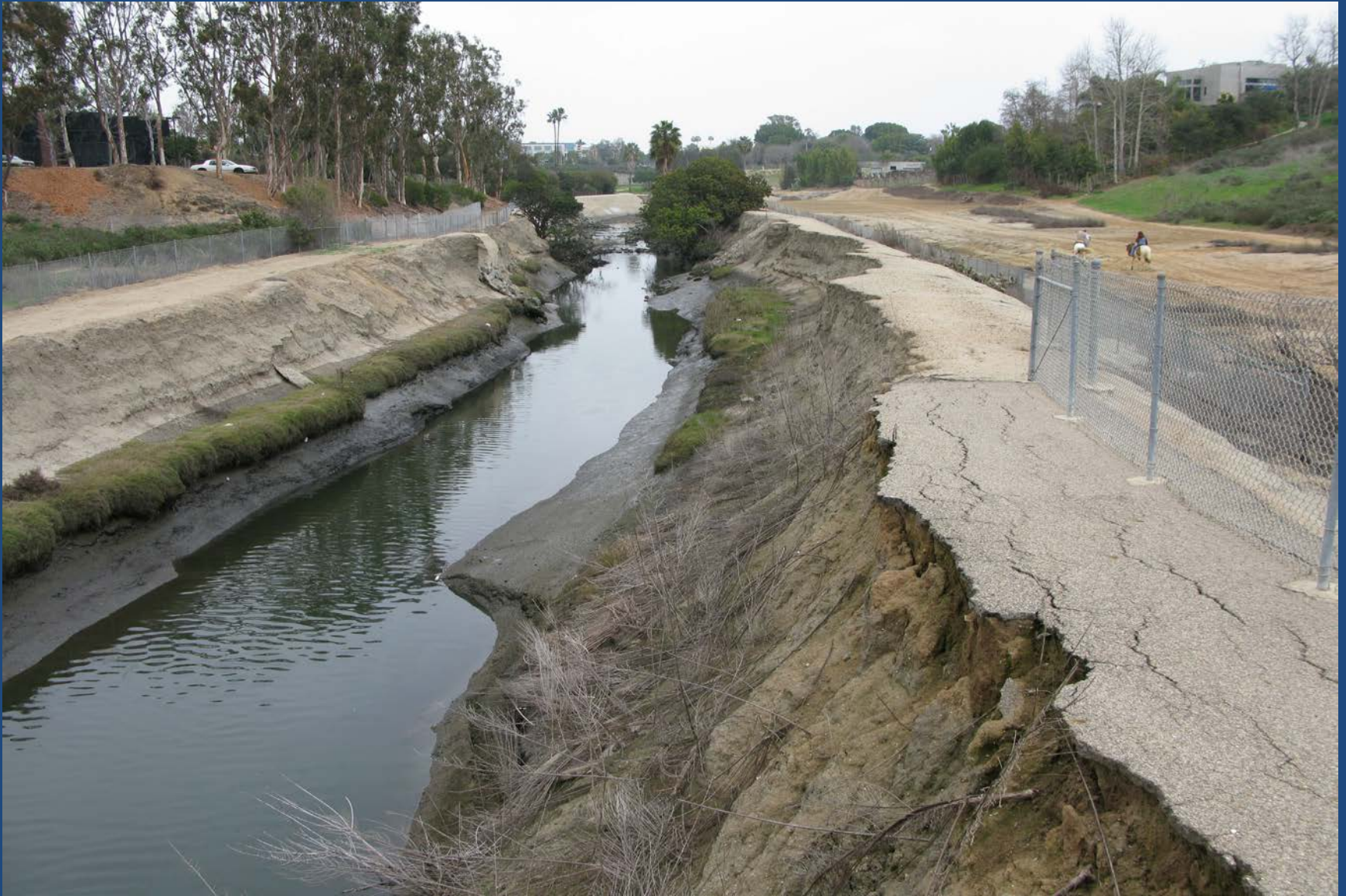
View Looking Upstream
