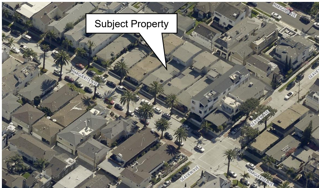
Figure 1: Oblique Aerial Image of Subject Property
