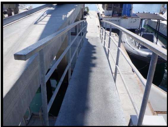
Boat Slip looking south, Hoist Platform to left
