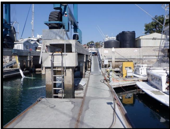
Looking north at property at water treatment tanks and hoist
