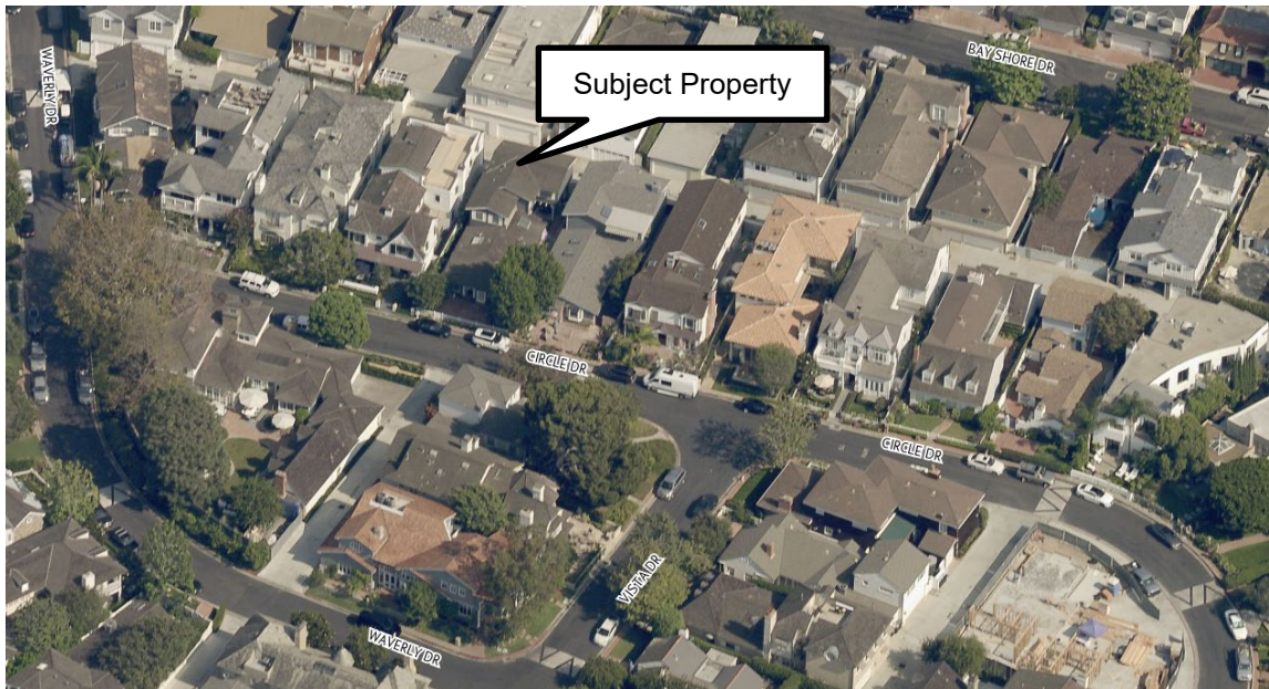
Figure 1: Oblique Aerial Image of Neighborhood
