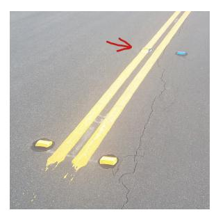
Additionally, in the follow-up a week or two later, that previous contractor seems to have misplaced either the striping or the reflectors, causing one to be painted over as shown at the arrow in the photo at left (and note more cracks to right of stripes).
