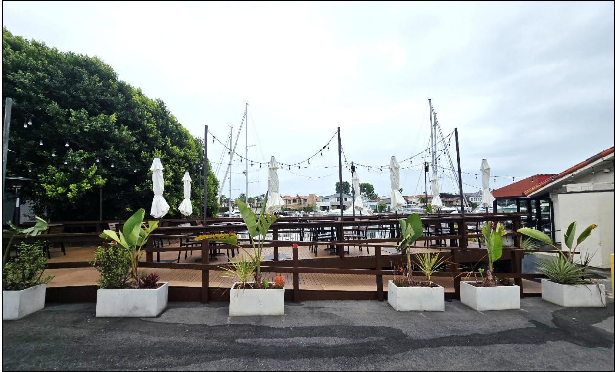
Figure 4, Existing Detached Patio with views towards Newport Harbor from the parking lot.
