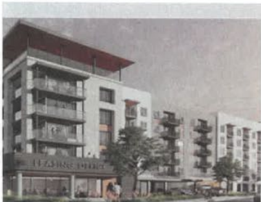
RESIDENCES AT 1600 DOVE STREET DEVELOPER: 1600 Dove St, LP and GS 1600 Dove ADDRESS: 1600 Dove Street PROJECT: Predevelopment stage. Proposal to demolish a 60,600-square-foot office to build a seven-story, 282-unit apartment (28 affordable units), podium style with parking on the first level
