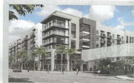
1400 BRISTOL RESIDENCES DEVELOPER: The Picerno Group ADDRESS: 1400 Bristol Street PROJECT: Five story 229-unit apartment (46 affordable), studio, one to two bedrooms
