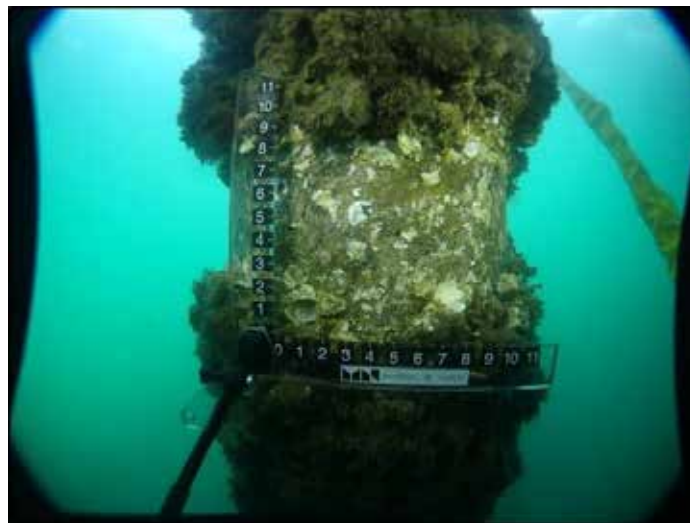
Photo 4-7: Typical timber pile condition under water (Level II inspection effort).
