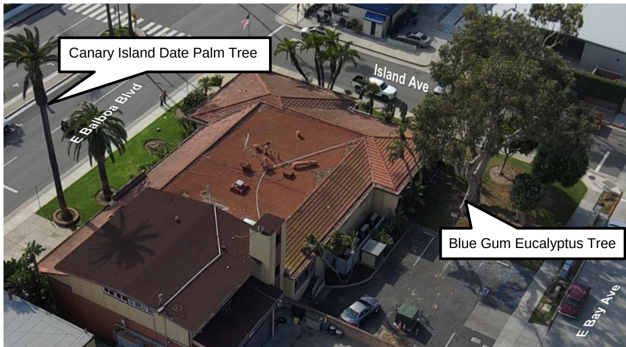
Figure 2: Oblique Aerial Image of Property
