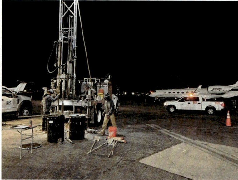
Photo 1: GMU conducting subsurface exploration to support ACI Jet redevelopment at John Wayne Airport.
