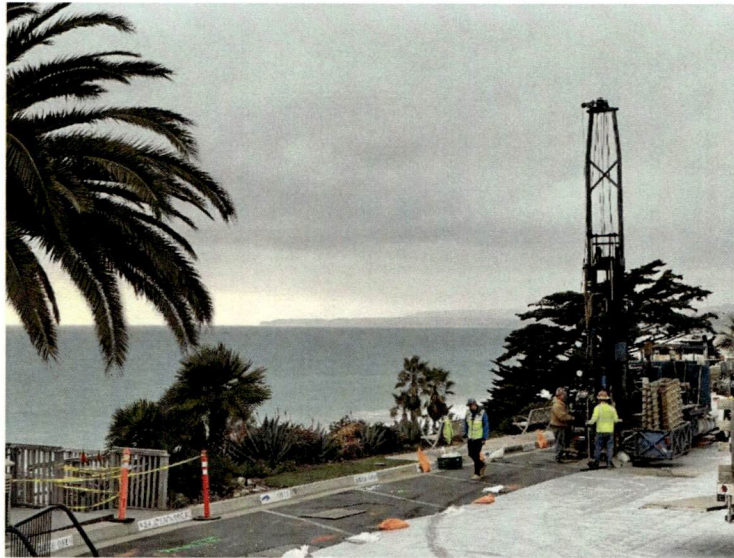
Photo 3: GMU conducting subsurface drilling for an emergency slope stability evaluation in San Clemente, California, along the bluff above the Metrolink rail line.
