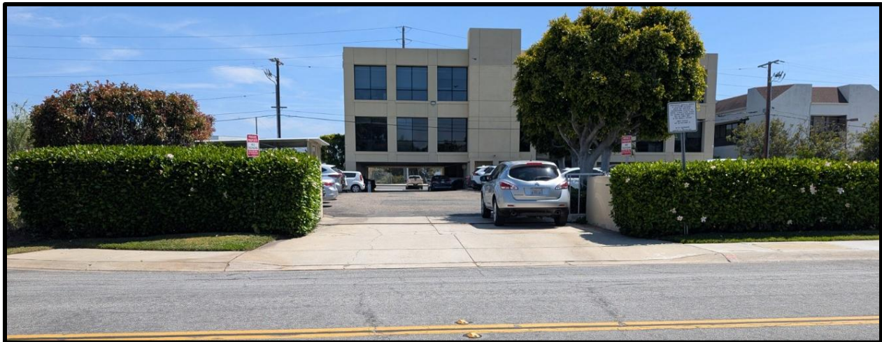
Figure 7, Photograph of existing Zenith Driveway condition with car entering
