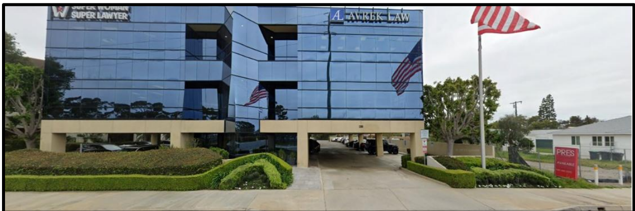
Figure 6, Google Street View image of existing driveway conditions from Bristol Street
