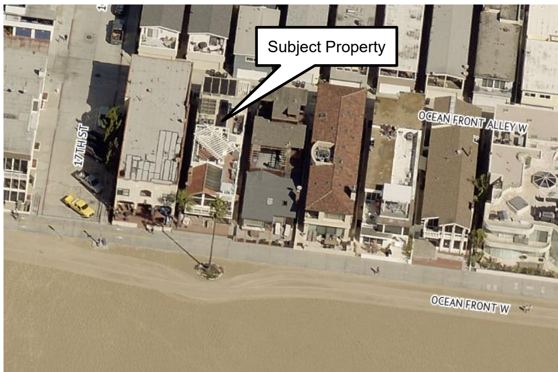
Figure 1: Oblique Aerial Image of Neighborhood
