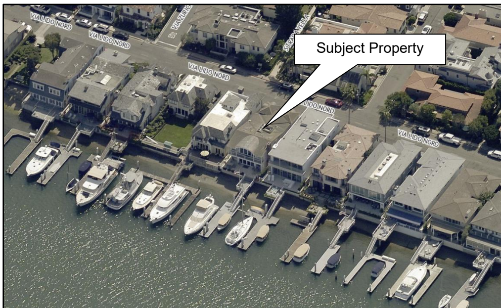
Figure 1: Oblique aerial image of neighborhood
