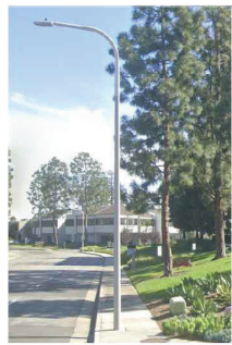
Existing Street Light
