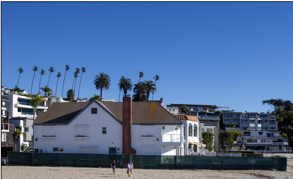
Figure 5: East elevation of existing residence from China Cove Street
