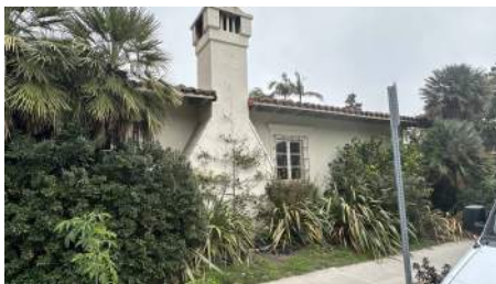
EXISTING BUILDING ALONG DAHLIA
