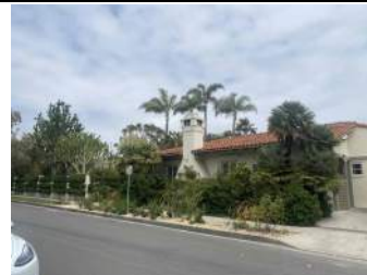
EXISTING BUILDING ALONG DAHLIA
