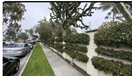
EXISTING WALL ALONG DAHLIA
