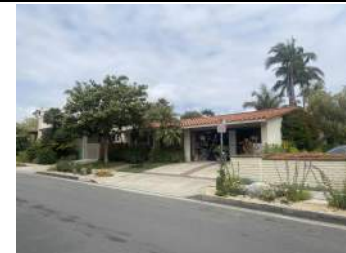
EXISTING BUILDING ALONG DAHLIA
