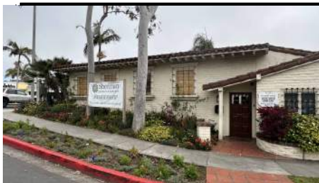
EXISTING BUILDING ALONG DAHLIA
