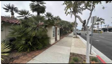
EXISTING BUILDING ALONG PCH
