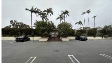
EXISTING BUILDING ALONG THIRD
