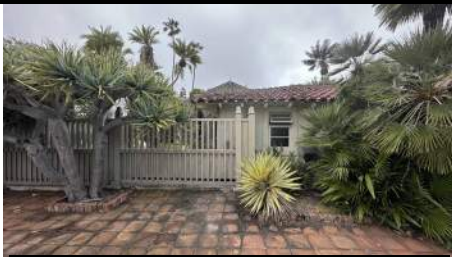
EXISTING BUILDING ALONG PCH
