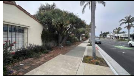
EXISTING BUILDING ALONG PCH
