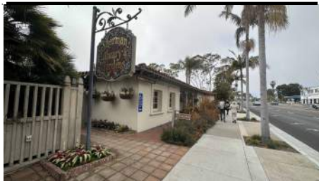
EXISTING BUILDING ALONG PCH
