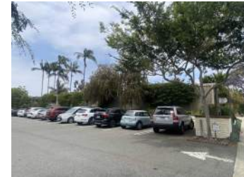
EXISTING BUILDING ALONG THIRD
