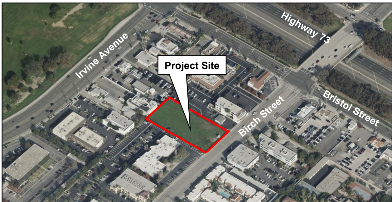
Figure 1, Oblique Aerial Image of Project Site and Vicinity.
