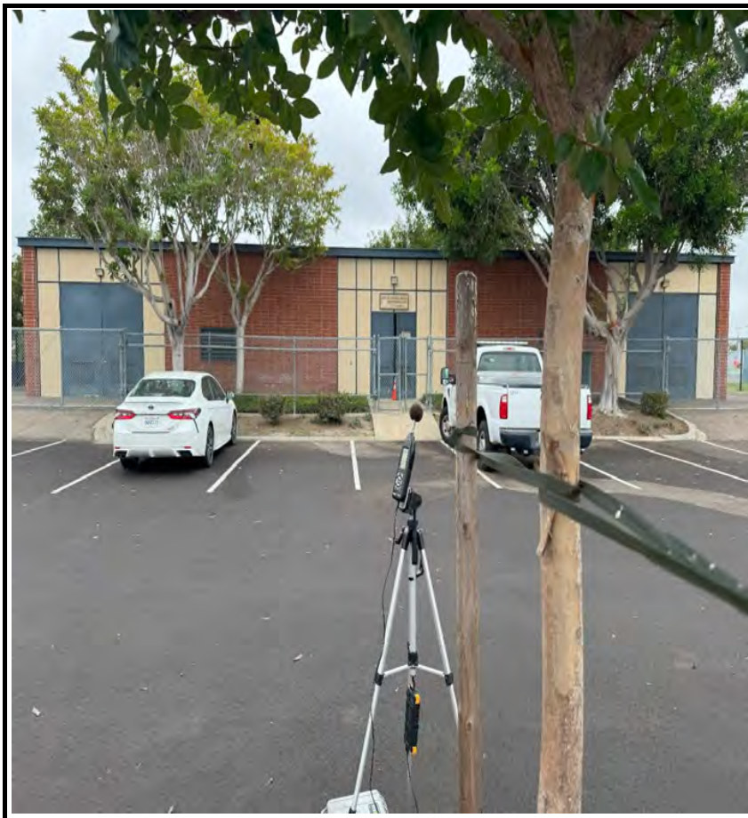
RNM1 looking W across parking lot towards main entrance to water well pump house 17399 Magnolia Street, Fountain valley ( 50' W ).
