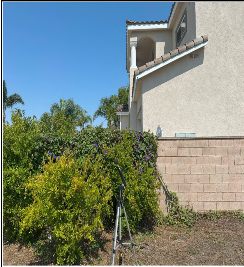
STNM1 looking E towards residence 9540 La Amapola Ave, Fountain Valley ( right ) & W end of La Amapola Ave behind 6' high vegetated chainlink fence (left ).
