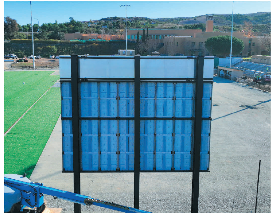
*EXISTING CONDITION - BACK OF SCOREBOARD
