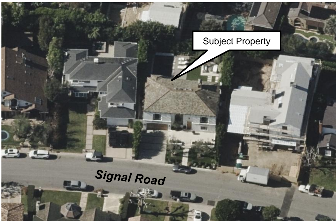
Figure 1: Oblique Aerial Image of Property
