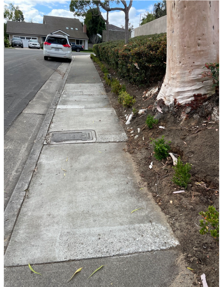
Photograph 4 – View of sidewalk replacement work as indicated by “newer” concrete.
