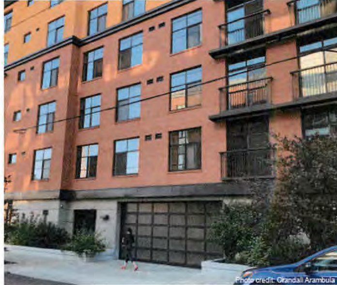
Parking structures shall be shielded from view from adjoining streets
