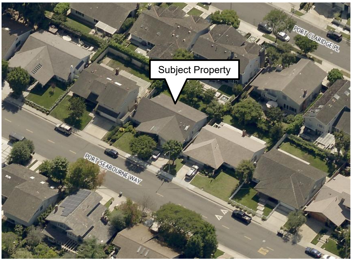
Figure 1: Oblique Aerial Image of Property
