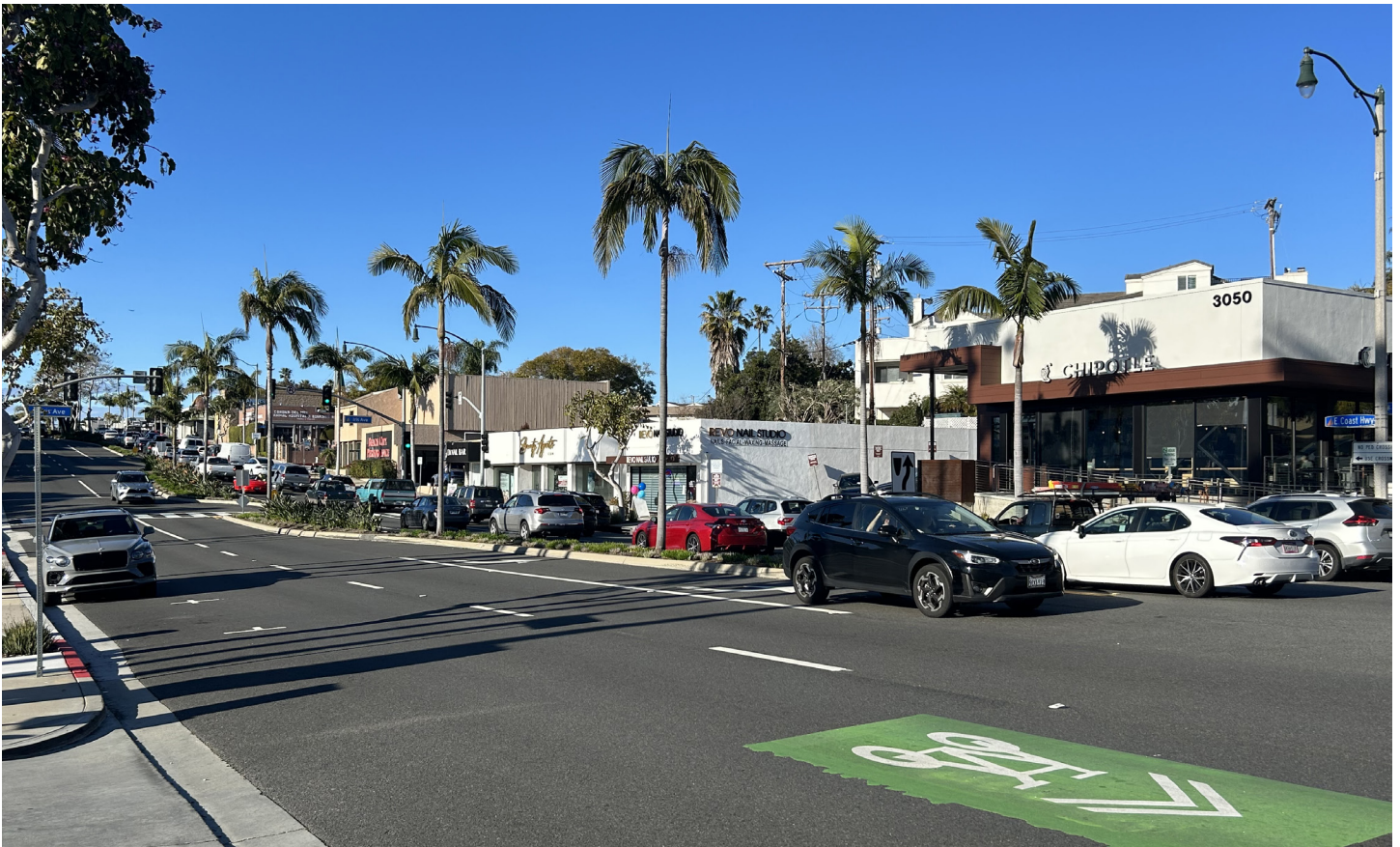
Existing Class III bicycle facility with sharrow pavement markings along Coast Highway
