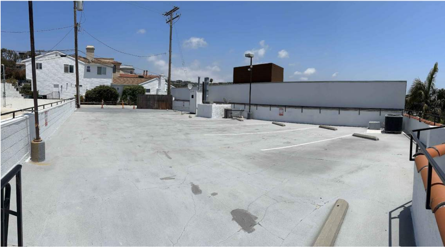
View of Roof from Stairs
