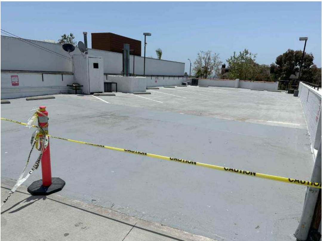
View of Roof from Alley
