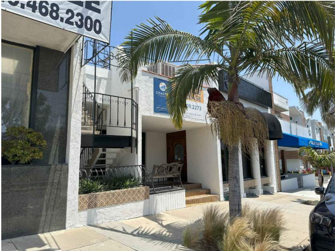
View from E. Coast Hwy Looking South
