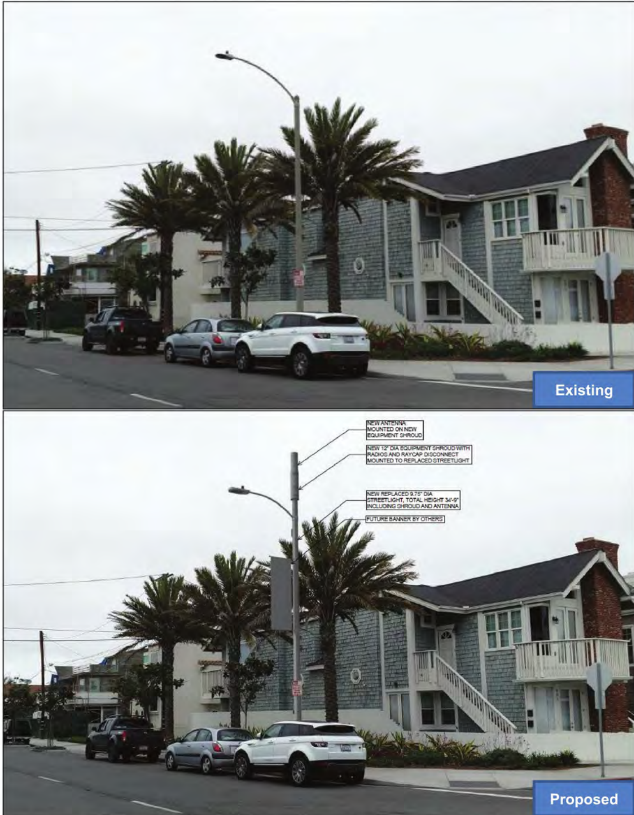
Figure 1, Existing photograph (top) with proposed rendering (bottom) showing the replaced streetlight pole, antenna, equipment shroud, and below-grade equipment handholes. The banner is only shown for reference and is not part of this proposal.
